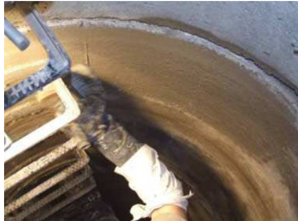
Photo 5: Sealing with crystallization mortar: backfilled annular gaps in the shaft wall (left); application as slurry coat with a wide brush (right)
