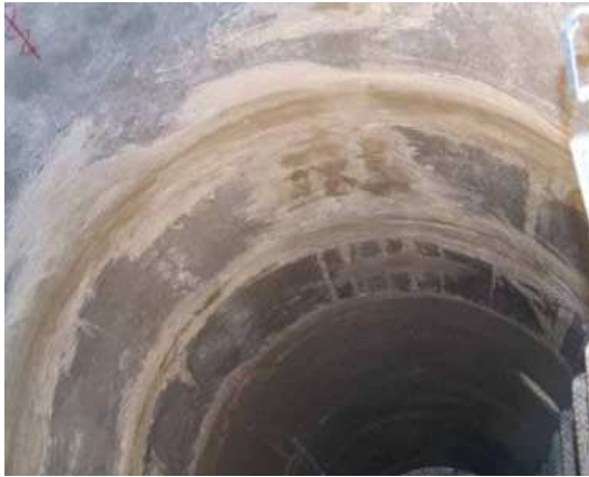
Photo 5: Sealing with crystallization mortar: backfilled annular gaps in the shaft wall (left); application as slurry coat with a wide brush (right)
